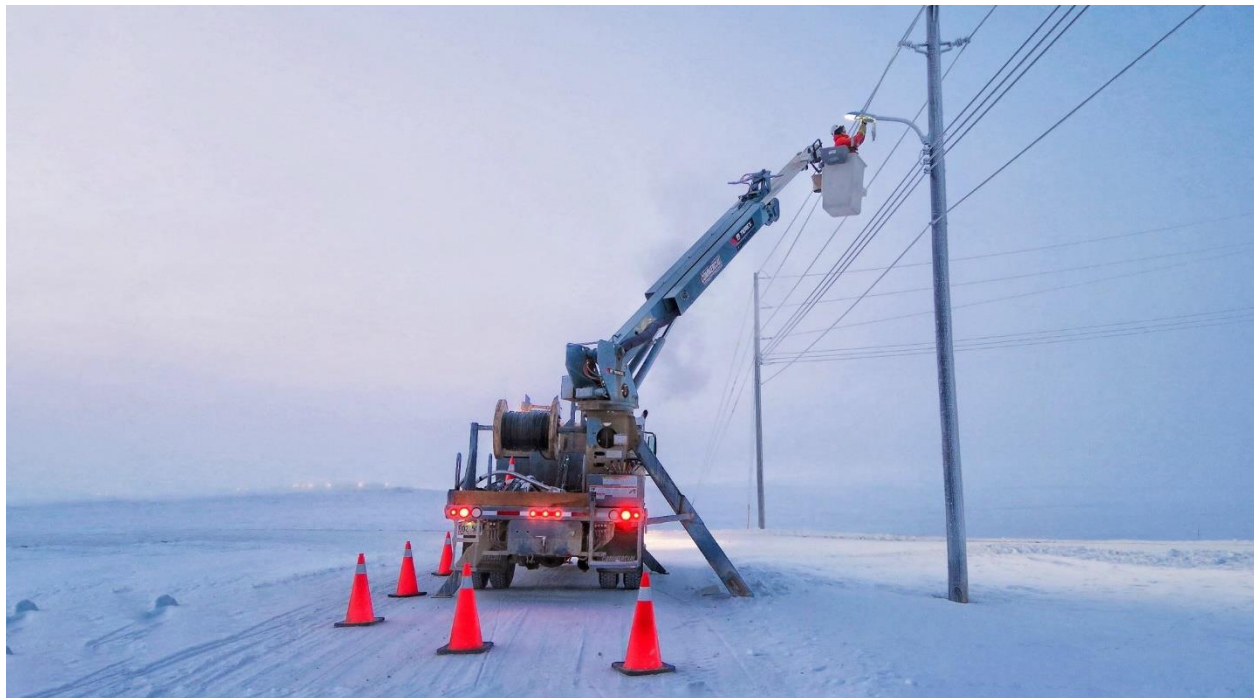
LED streetlight installation
