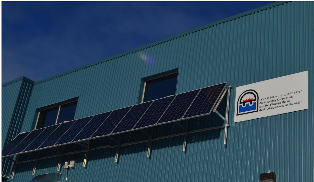
Solar panel installation at Iqaluit power plant
